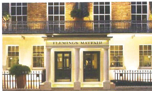
Fleming's Mayfair is undergoing a £2 million two-phase refurbishment
